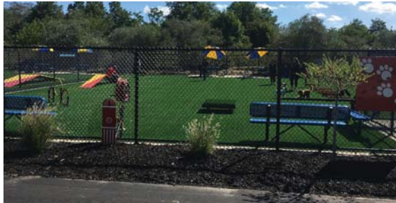
1 6' Chain Link Fence set in Concrete
