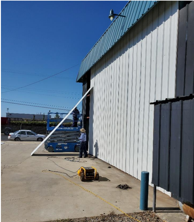
Facilities Maintenance staff installed new metal panels at 79 N Sunnyside.
