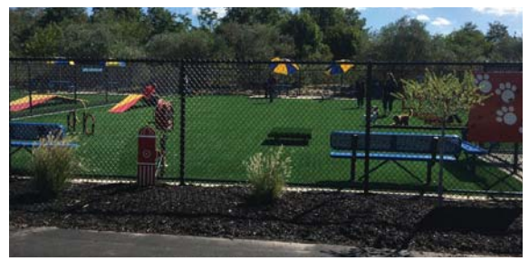
6 6' Chain Link Fence set in Concrete
